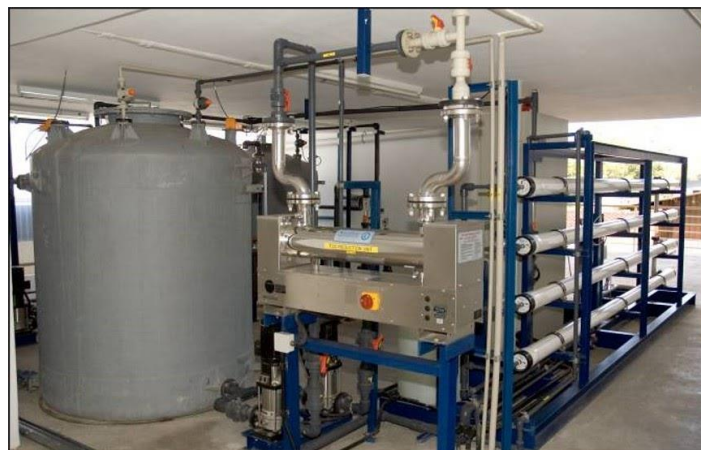
DI Water Recovery: DI Water Recovery System Photo
